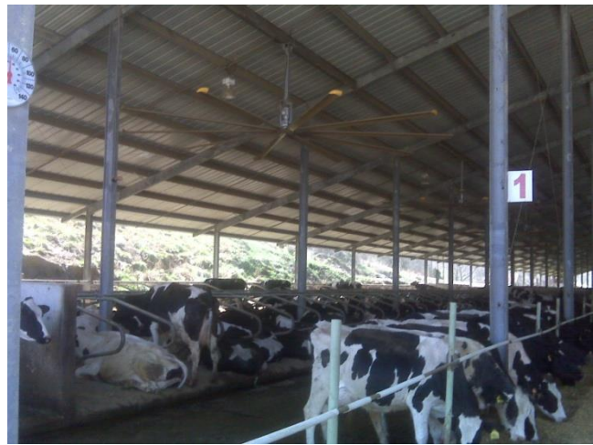
Figure 25. The ideal freestall barn maximizes natural ventilation with high, open sidewalls, a ridge vent opening and supplements natural ventilation with fans used to increase air flow and exchange.
